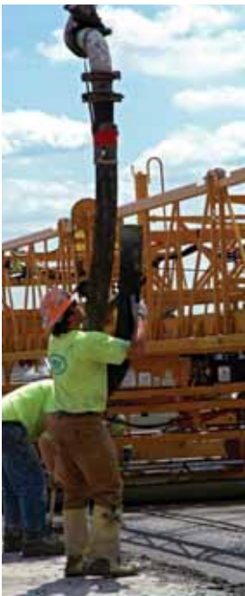
Workers operate concrete pump in the building of the I-94 Business loop of Memorial Bridge in North Dakota. Photo courtesy of Mike Kopp, North Dakota Department of Transportation, 2008.
